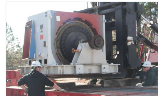
The pumphouse motor is safely placed on a lowboy trailer.
