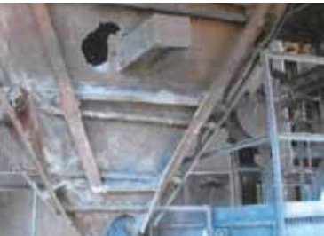
Before (Left) and after (Below) the damaged precipitator hopper was repaired.
