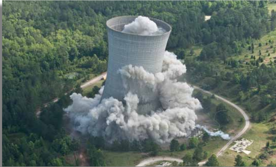
K Cooling Tower was one of seven industrial buildings demolished.
