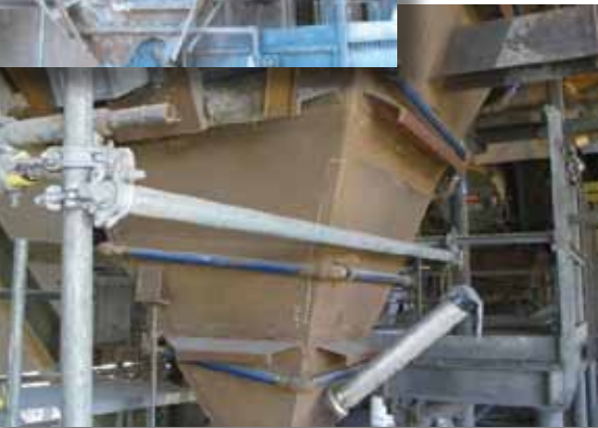
Before (Left) and after (Below) the damaged precipitator hopper was repaired.
