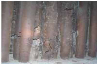
Before (Left) and after (Below) the deteriorated pre-heater tubes were replaced.
