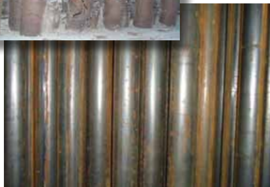
Before (Left) and after (Below) the deteriorated pre-heater tubes were replaced.
