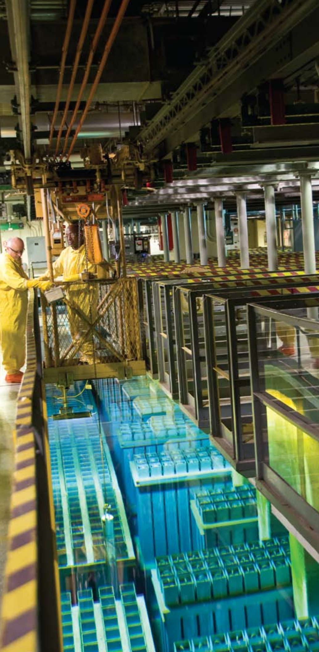
Transporting a fuel bundle to its storage location in the L Area Complex
