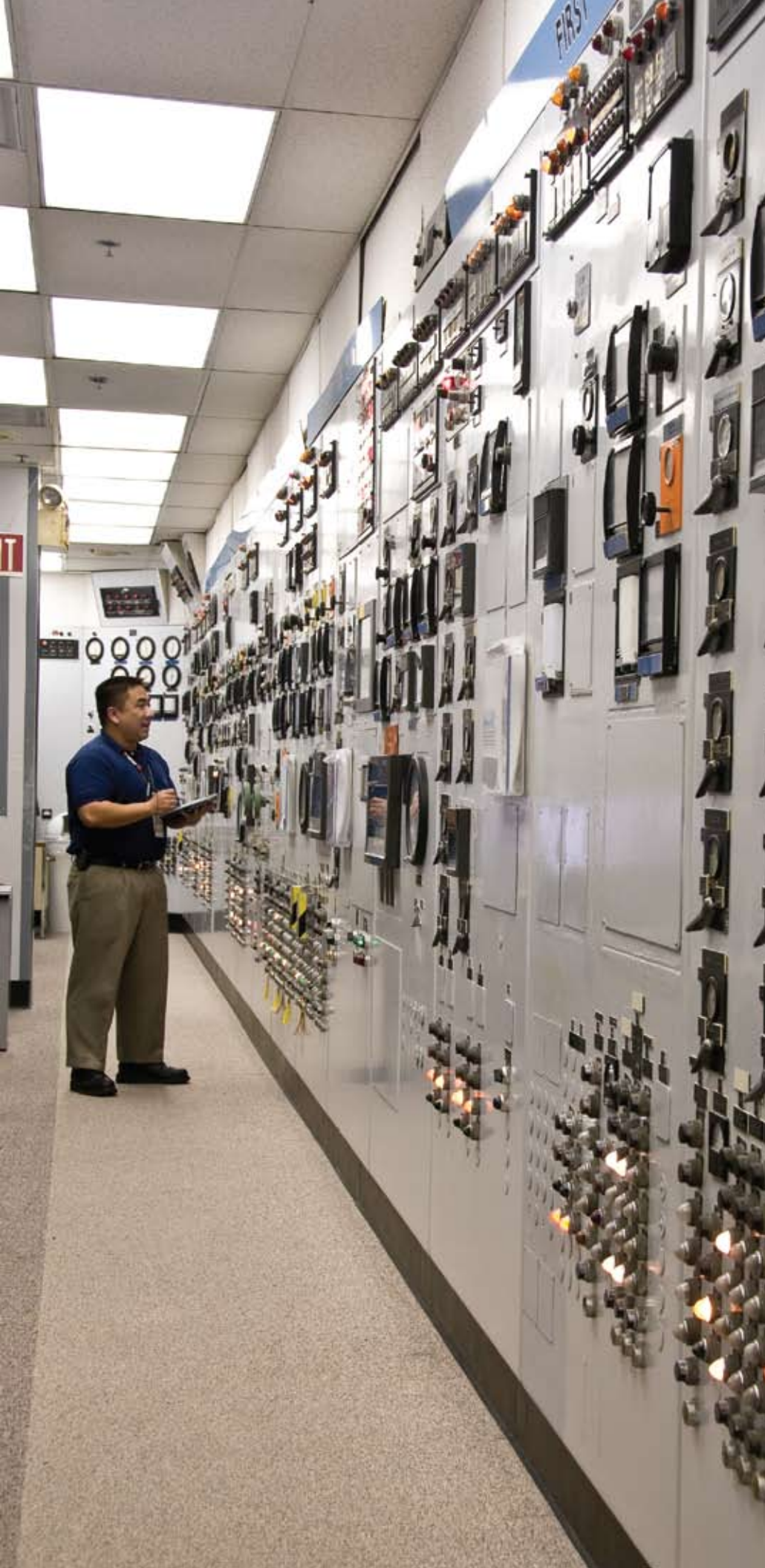
Reviewing process roundsheet readings in the H Canyon control room
