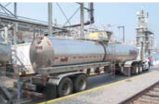
Unloading a chemical shipment from a tanker truck into a storage tank in the H Canyon Outside Facilities
