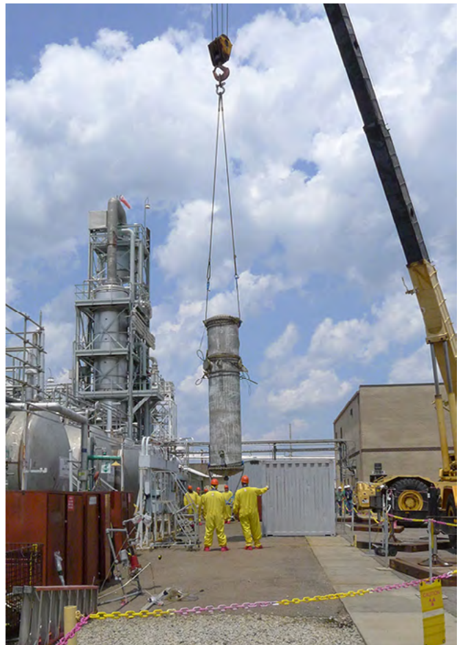
A crane operator lowers the old reboiler from the Acid Recover Unit to allow workers to attach it to a second crane in preparation for final storage. Replacing the 8,500 pound component required a complex process.
