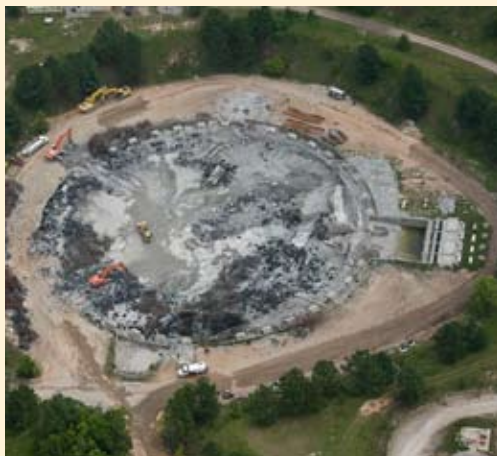
SRS Recovery Act workers (above) used heavy equipment to remove the rubble of K Cooling Tower while sorting more than 800 tons of reinforced steel for recycling. (At right) K Cooling Tower was imploded on May 26, 2010 as part of the SRS Recovery Act Project.
