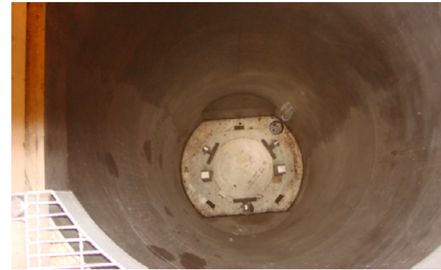
The Adaptor Plate at the bottom of the Shielded Transfer System helps align the cask into the system.
