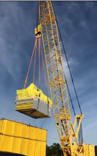
A crane lifts the HAWTT from containment to place on the railcar.
