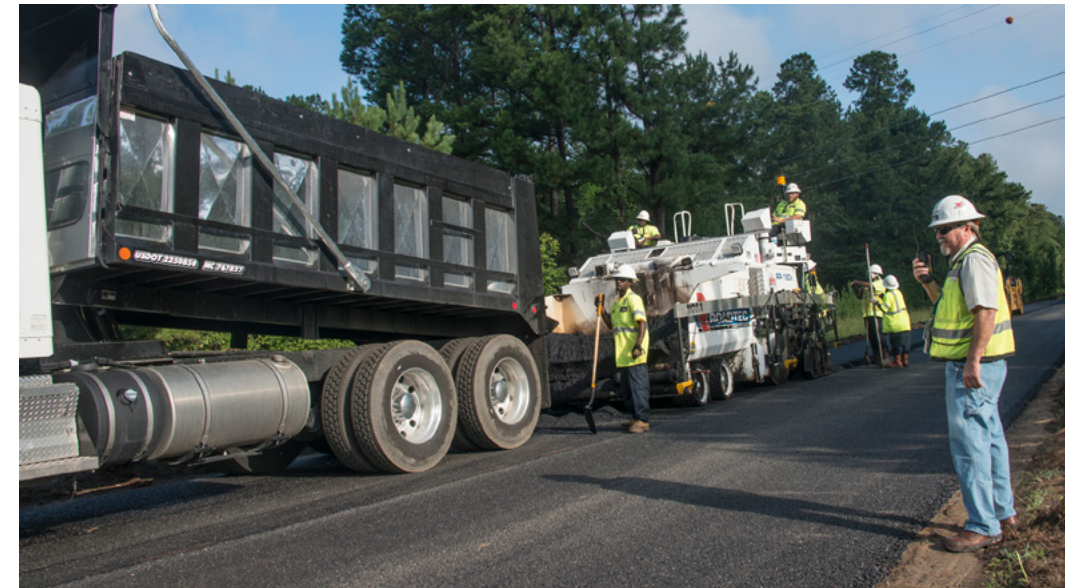
Wayne Cadden, SRNS Subcontract Technical Representative, monitors the progress of a new, highly cost-effective method to resurface cracked, aging roads found at several SRS locations.
