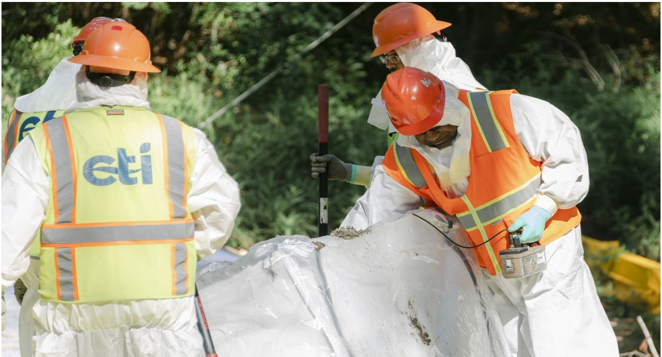
CTI personnel remove contaminated sediment from the R-Reactor Discharge Canal at Savannah River Site.
