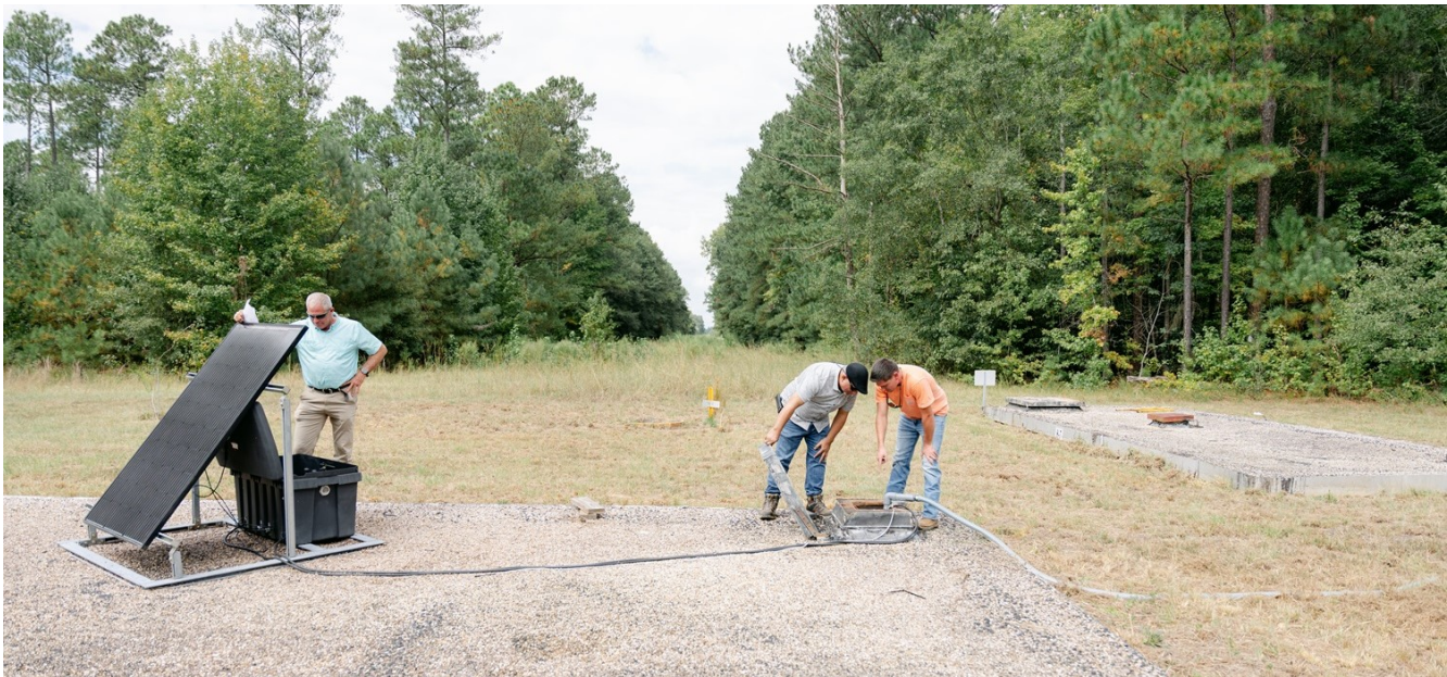
Savannah River Nuclear Solutions (SRNS) Site Services Billy Vowell, Water Operator; Rich Brown, Engineer; and Tyler Handberry, Water Operator, inspect the D Area solar-powered pump system that manages water infiltration in underground valve pits at the Savannah River Site.
