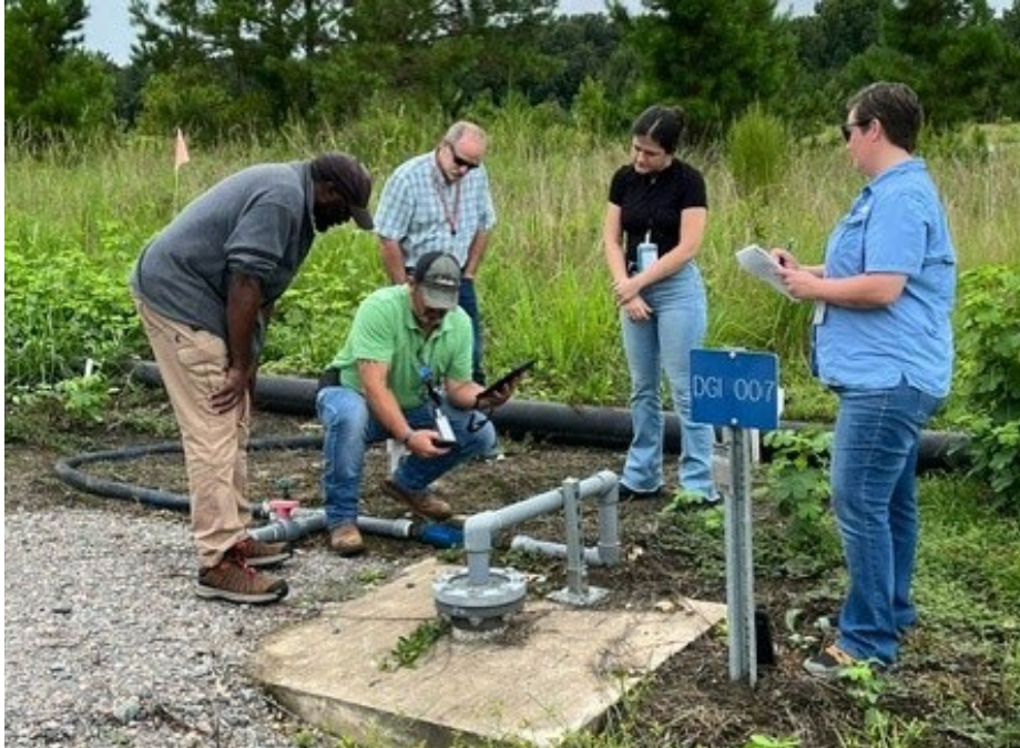
D Area Groundwater Treatability Study project team assesses artesian flow into injection well.
