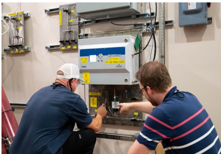
SRTE Carson Blake and Chadwich Mattox perform functional checks on a newly installed Glovebox Oxygen Monitor.
