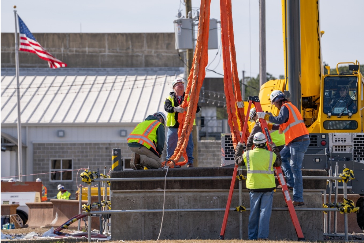
Personnel installed the appropriate rigging needed to lift the 41,000-pound hatch.
