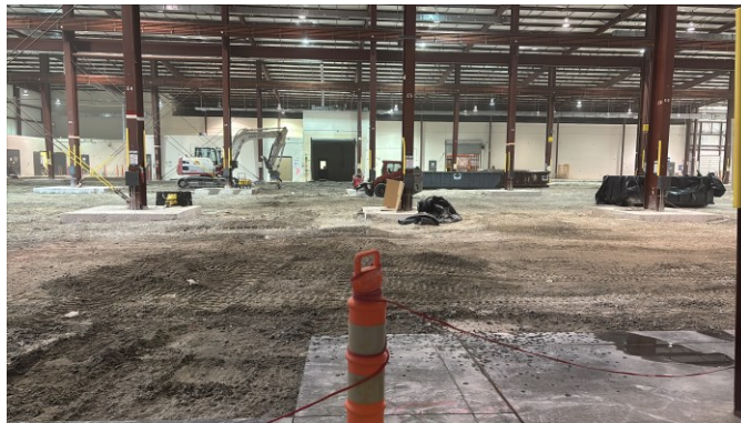
Floor removal operations within the HFTOC
