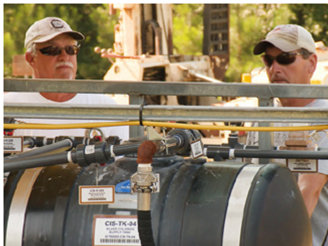
SRNS operators Stanley Creech (left) and Paul Dobson monitor the injection of silver chloride into the aquifer beneath F Area at the Savannah River Site. Results of a recent test indicate a significant decrease in the hazard posed by contaminants where silver chloride was injected.
