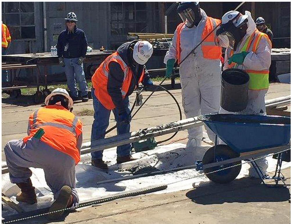
*SRNS Construction workers placing concrete into a thermowell for an H Area project.*
