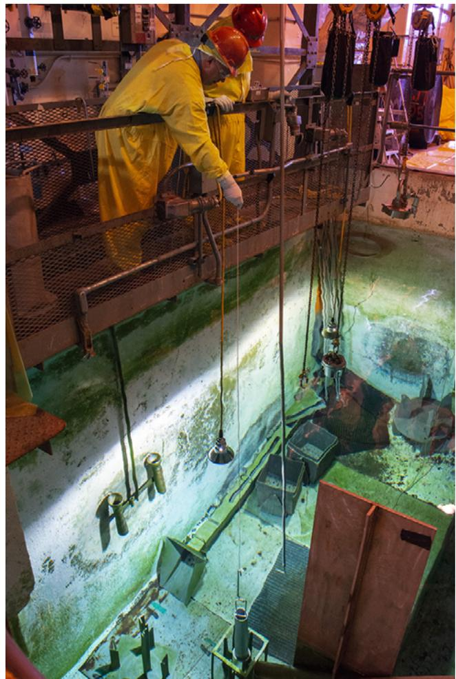
*SRNS Operators, whose work contributes to SRNS’ achievement of 25 Million safe-work hours, prepare the GE-2000 spent nuclear fuel shipping cask to be safely lifted out of its base by an 85-Ton Crane.*
