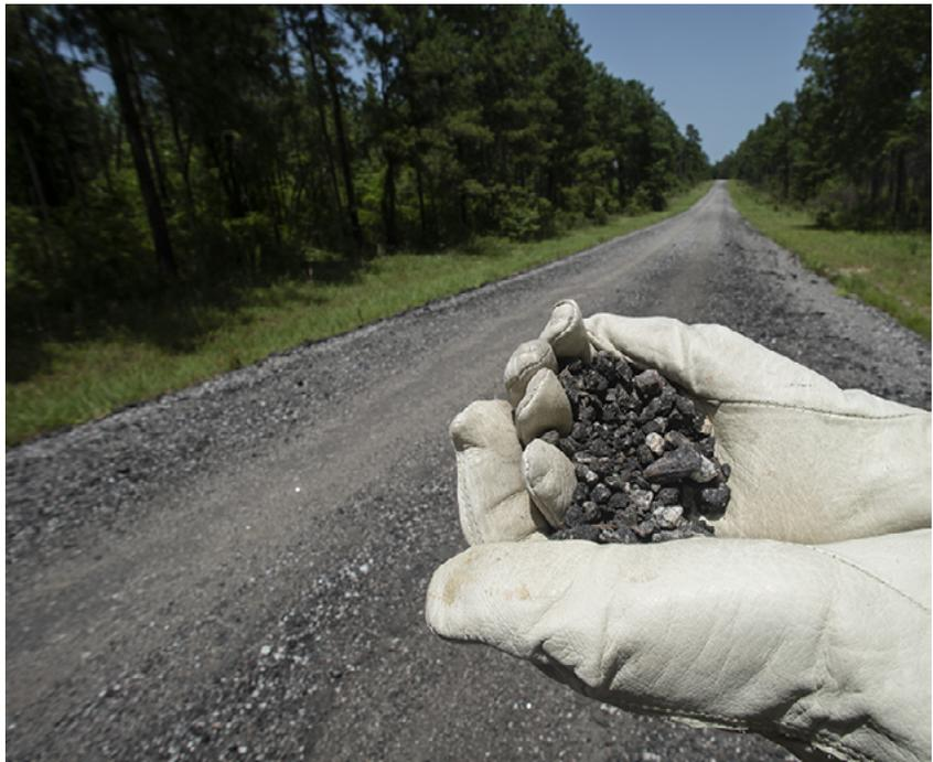
*SRNS reuses road millings to resurface secondary roads at SRS and in Orangeburg County, furthering the lifecycle of Site resources and reducing waste.*
