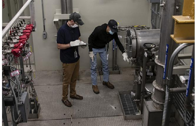
*Operator apprentices Adam Thomas and Chadwick Champy making operator rounds and recording pressure gauge readings*
