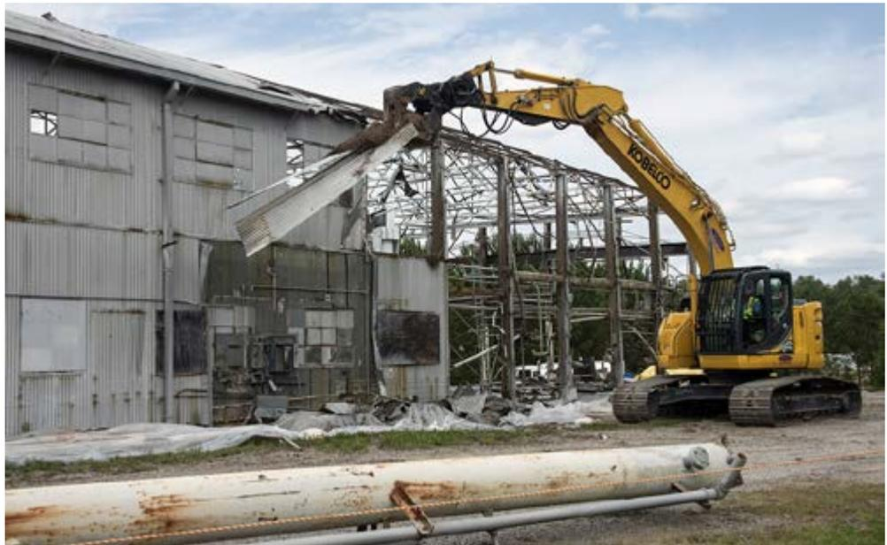
*At the height of the Cold War, the Ford Building was used to test components used in five nuclear reactors at the Savannah River Site. An excavator is shown here removing a section of the facility's metal roof.*
