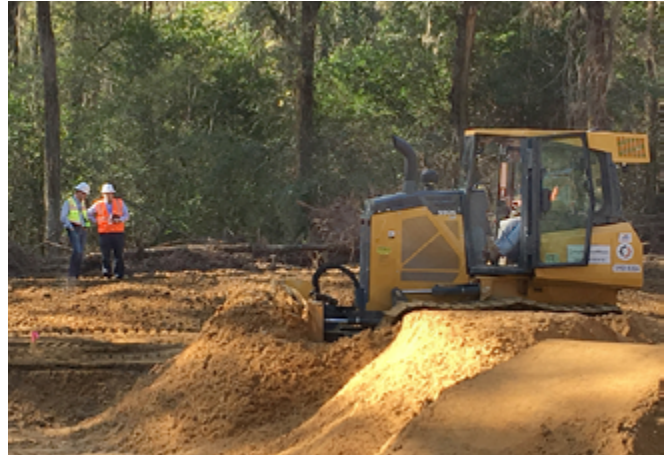
Savannah River Nuclear Solutions engineers Justin Fuller, left, and Steve Conner evaluate progress in the cleanup of a pond-like basin containing low levels of herbicides and pesticides at the Savannah River Site.
