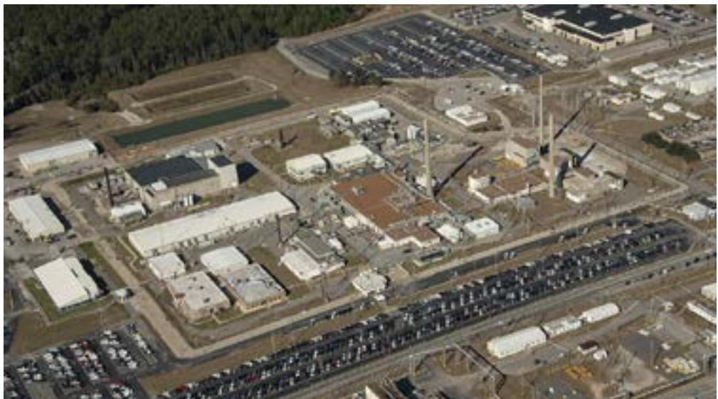
Aerial of the tritium facilities at SRS
