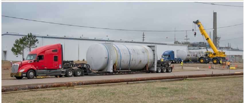
Cranes loaded the generators and tanks onto their trailers, in precise operations overseen by safety observers.
