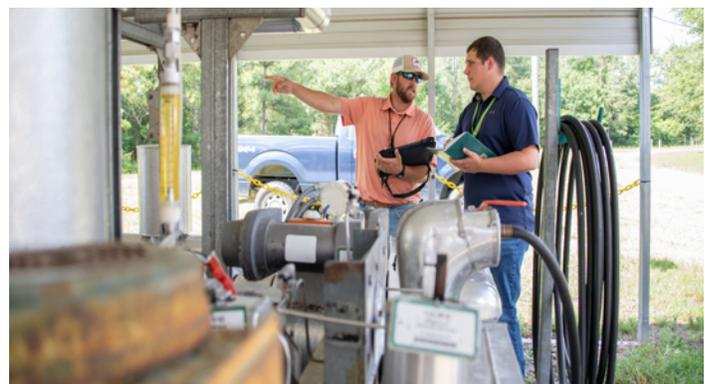
*F Area Operator Thomas Harman (left) and SRNS Scientist Kevin Boerstler check the pumps, sensors, and piping that blend a base concentrate to inject into acidic groundwater at SRS, part of the Site's environmental remediation strategy.*
