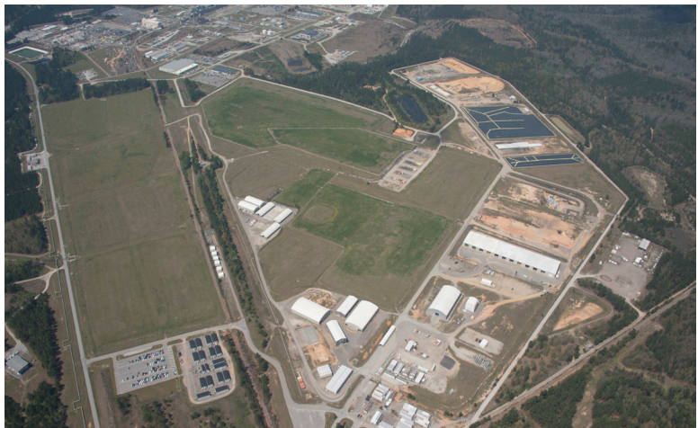
The Solid Waste Management Facility at SRS.
