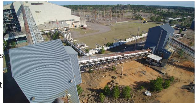
*In past Savannah River Site operations, a coal handling system in the site's D Area delivered coal to the top of the D Area Powerhouse where it was burned to produce power and steam. Workers have demolished the system's conveyors and associated buildings pictured here in gray. The site provided salvaged conveyor belts to the nonprofit Savannah River Community Resource Organization for beneficial reuse in the community.*
