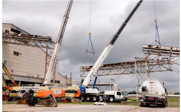
*SRS workers dismantle the conveyors of a coal handling system in D Area. Multiple structures from the coal transfer system plus three small support buildings were demolished creating nearly 84,000 cubic feet of metal, which has been relocated to a salvage site for recycling.*
