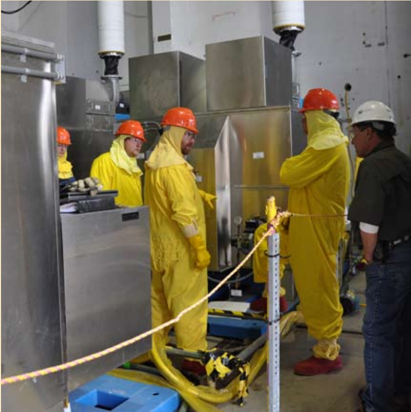
SRNS radiological workers run clean water through the evaporators in the Transfer Bay at the P Reactor Disassembly Basin as part of testing for evaporator startup.
