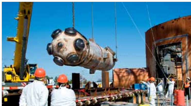
(Above) SRS removes one of the two 41,600-pound steam generators that were designed to cool HWCTR. (Below) The generator is leveled horizontally after coming out of the top of the reactor building. The generators will be transported to the Site's burial ground for disposal.
