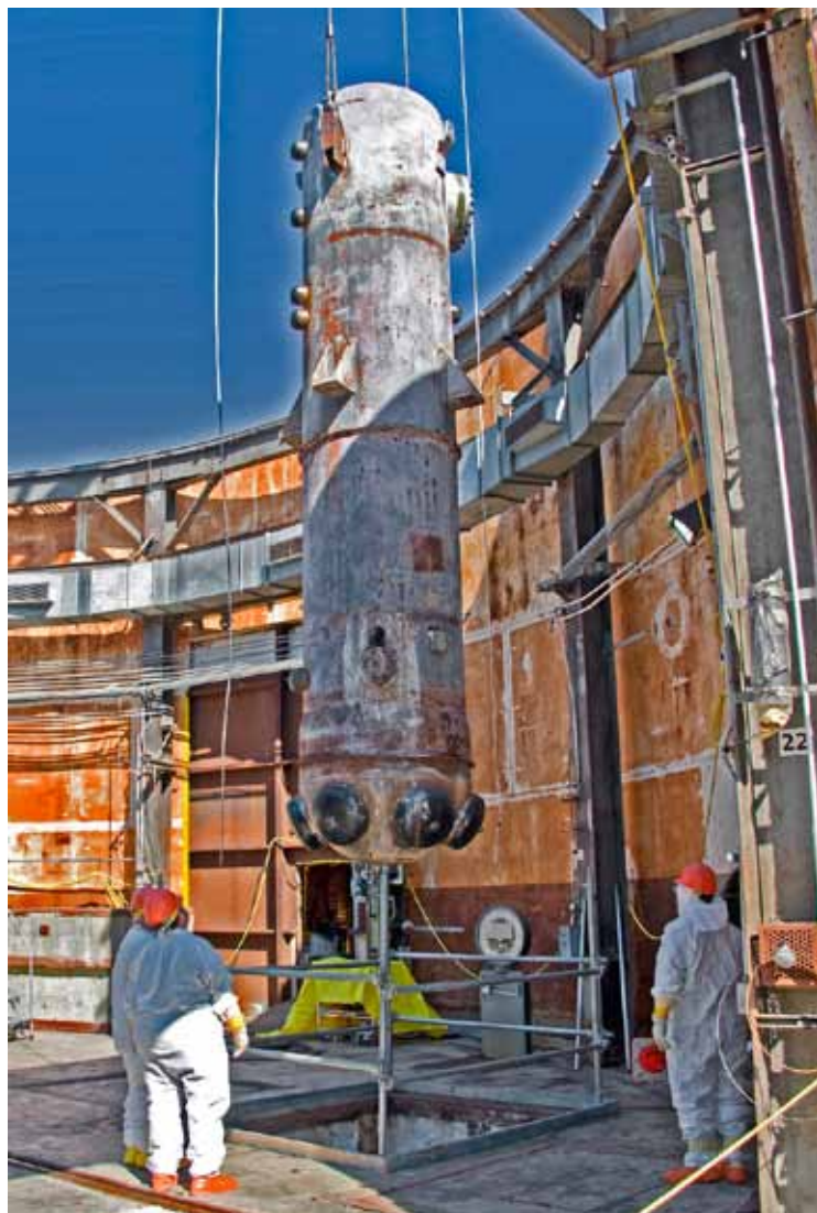
(Above) SRS removes one of the two 41,600-pound steam generators that were designed to cool HWCTR. (Below) The generator is leveled horizontally after coming out of the top of the reactor building. The generators will be transported to the Site's burial ground for disposal.
