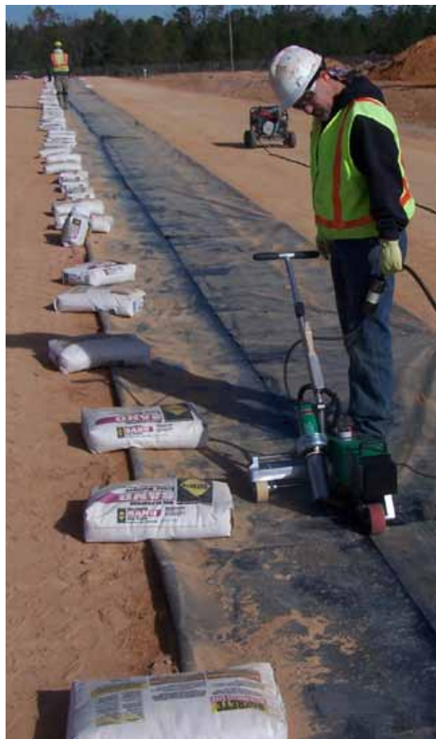
The liner installer heat-welds a sand anchor closed. The sand anchors are installed under the liner and across the length of the slit trench to keep the liner in place and minimize the effects of wind lift.
