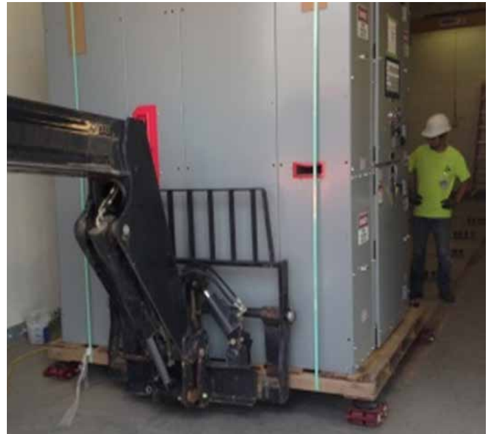
A new 13.8kV switchgear has been installed in 151-1L.
